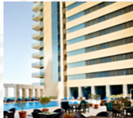
ASAS TWIN TOWER
